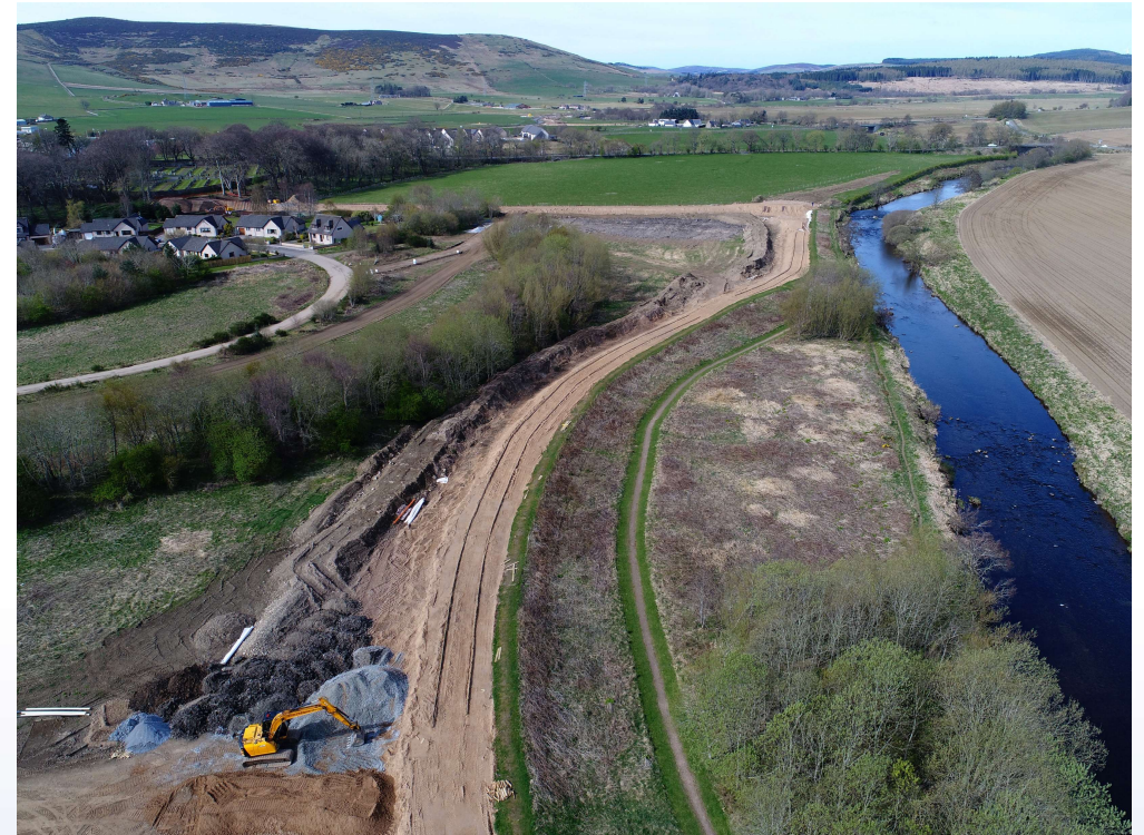
Huntly – Rural, large scale earthworks
